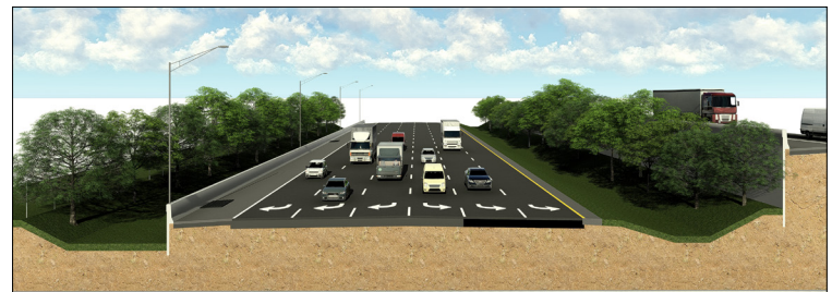
I-95 southbound exit ramp - Widening from 4 existing lanes to 6 proposed lanes
